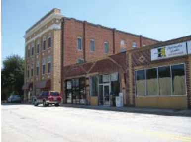
Storefronts within the downtown
