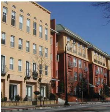
Multi-family housing is recommended along Thompson / Dorsey Streets
