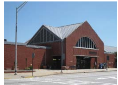
The East Point MARTA Station
