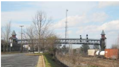
Pedestrian Bridge near the East Point MARTA Station is an iconic feature in the downtown
