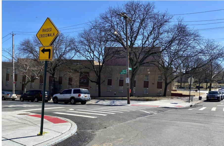
Figure: Raised Crosswalk at Intersection
