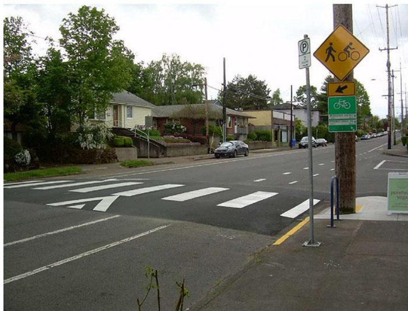
Figure: Raised Crosswalk at Mid-Block
