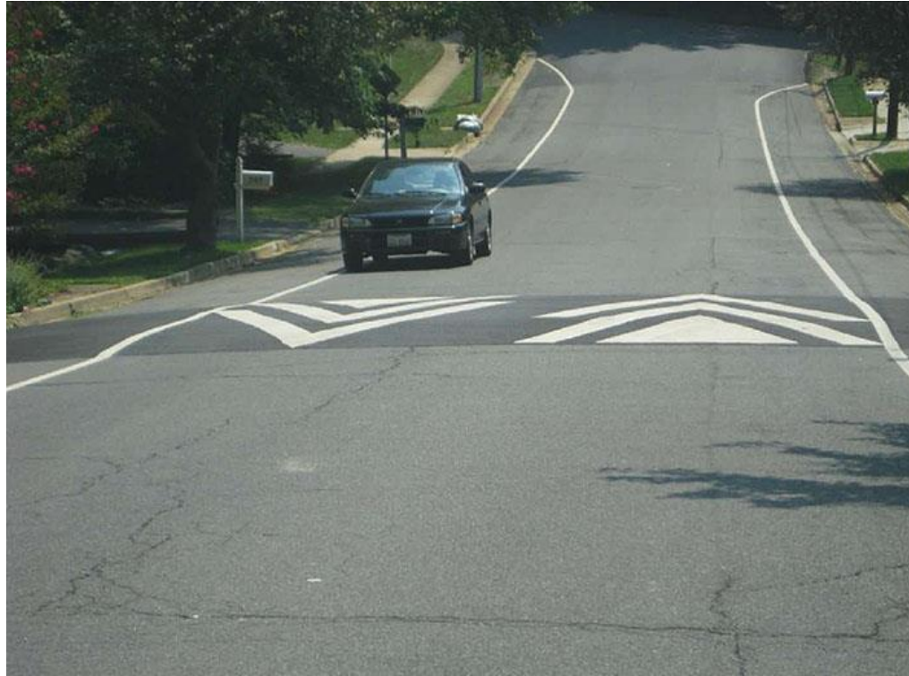
Figure: Example of Speed Hump
