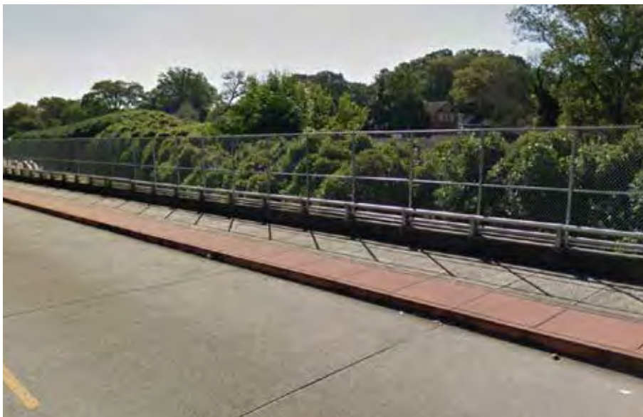
A modified bridge on Westview Dr SW in Atlanta to accommodate a 10' wide multi-use trail
