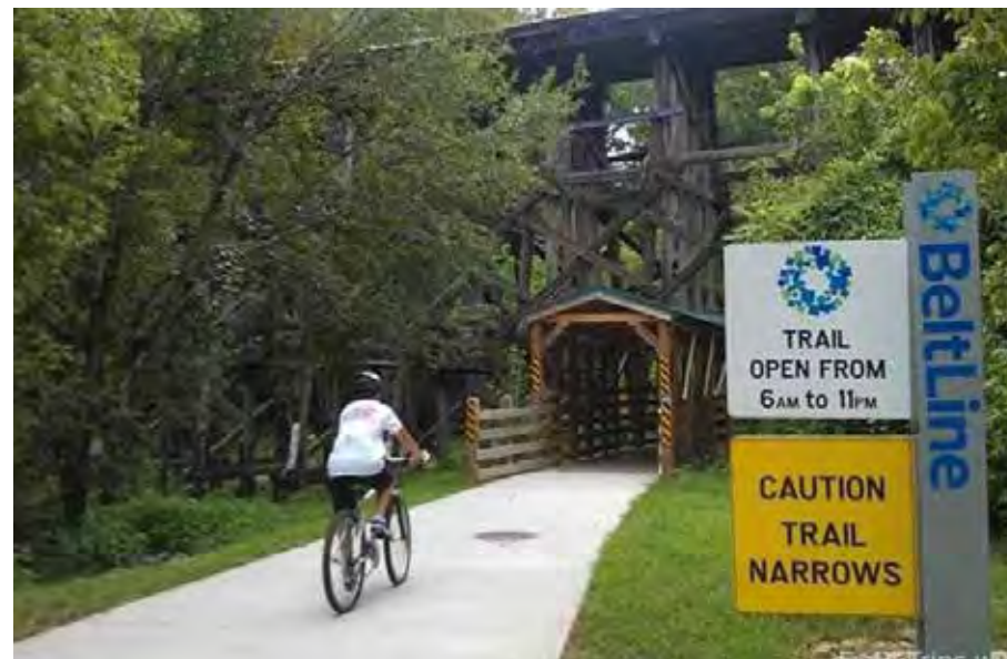
Canopy protective structure over trail when going beneath railroads.
