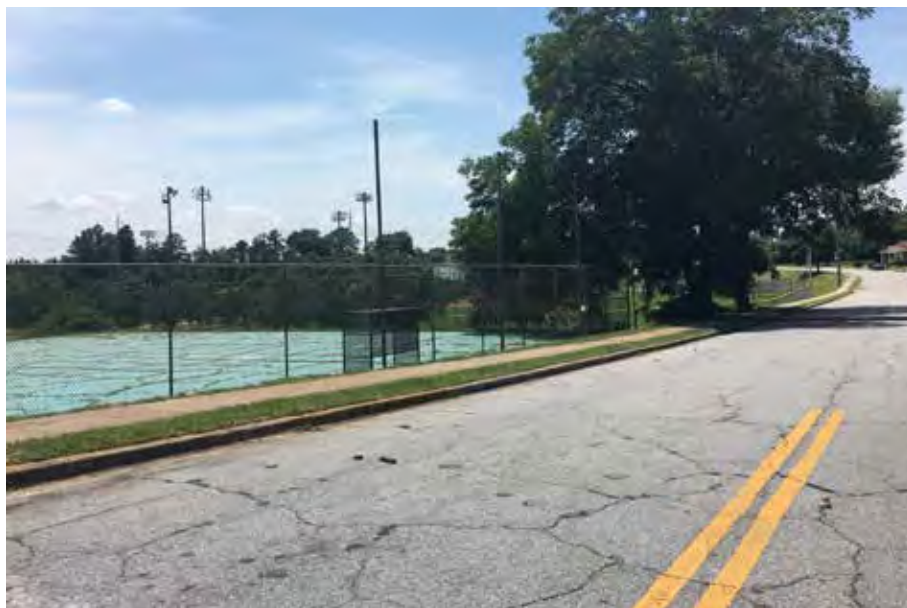
Existing conditions of John D. Milner Athletic Complex on Martin St
